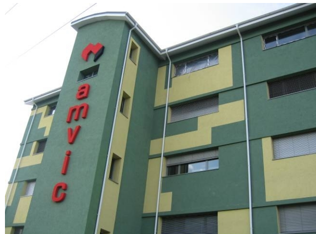
Fig.2 – Facade of Amvic Building
