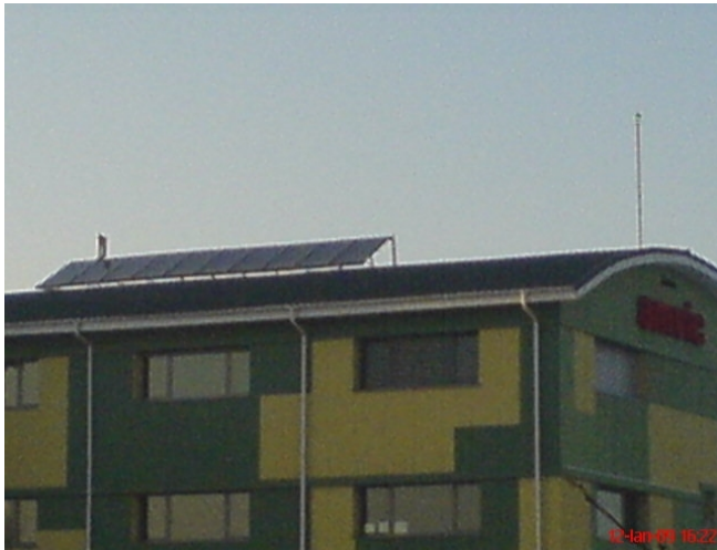
Fig.4 – Solar vacuum installation on Amvic Building
