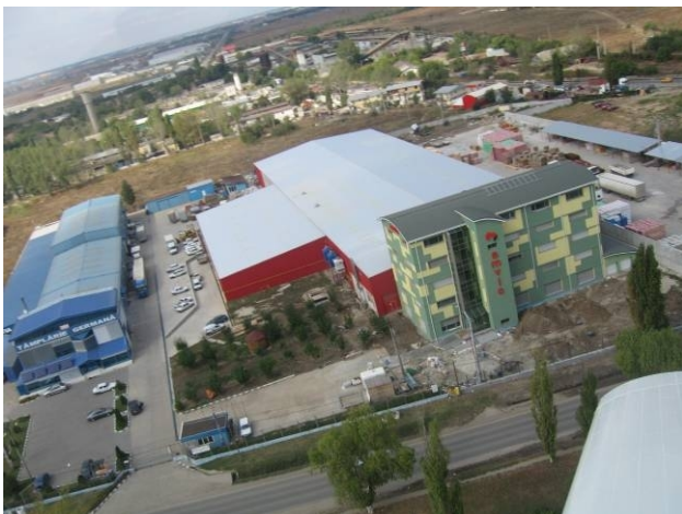
Fig.1 – Plain view of Amvic Building
