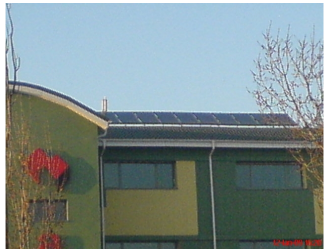
Fig.5 – Solar vacuum panels on the roof
