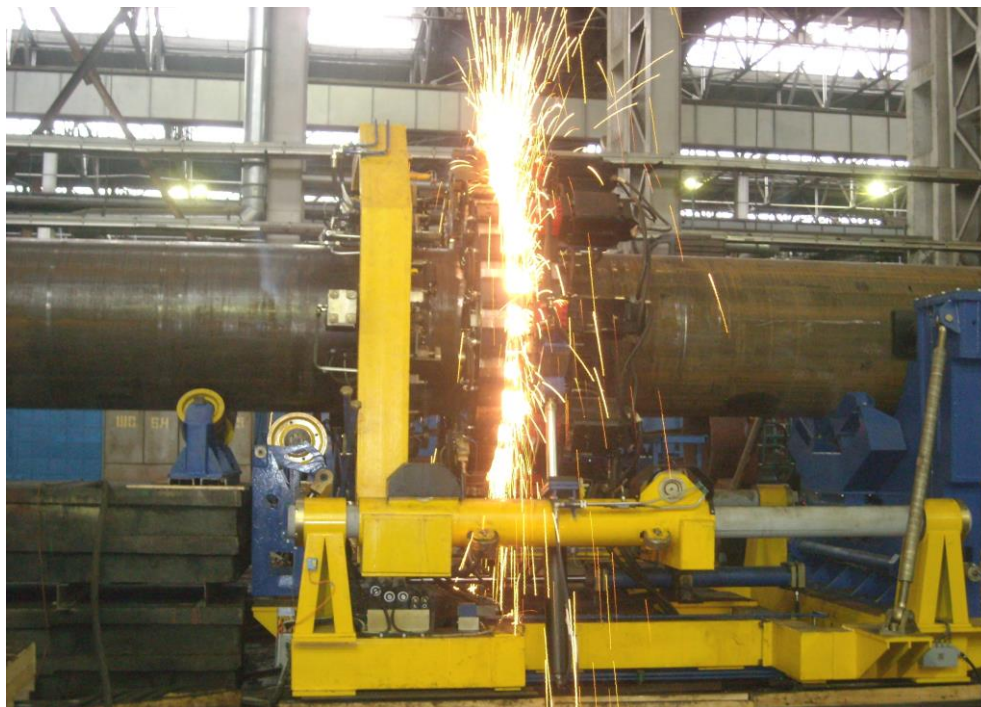
fig.2b. Second generation external 48 inch FBW machine during welding
