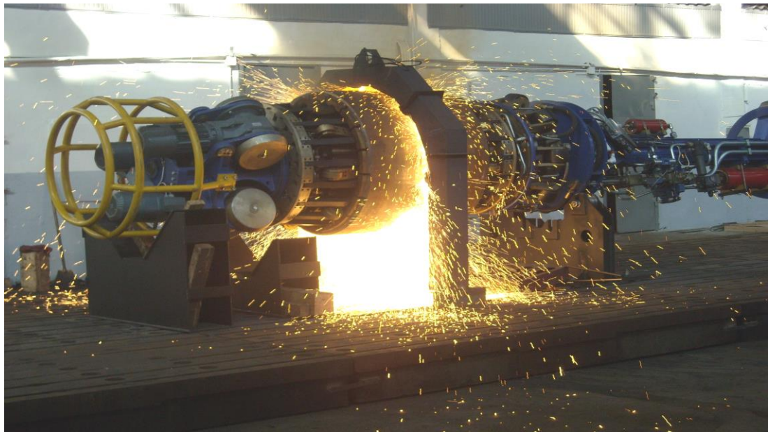
fig.1b. Second generation internal 48 inch FBW machine during welding
